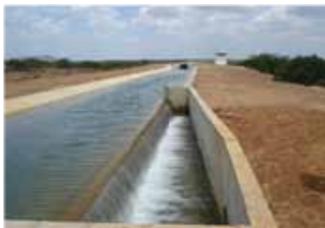
Canal Principal e Extravasor
